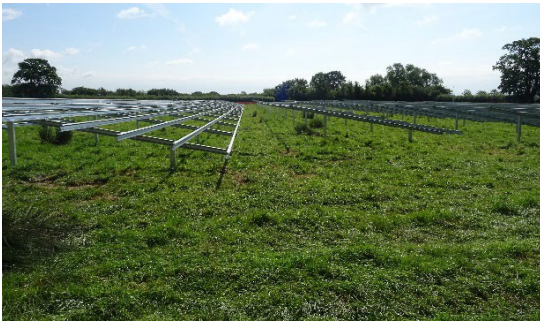
Inserts 28 and 29: Ground After Construction
