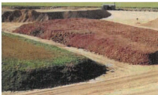
Clearly defined stockpiling of different soil materials
