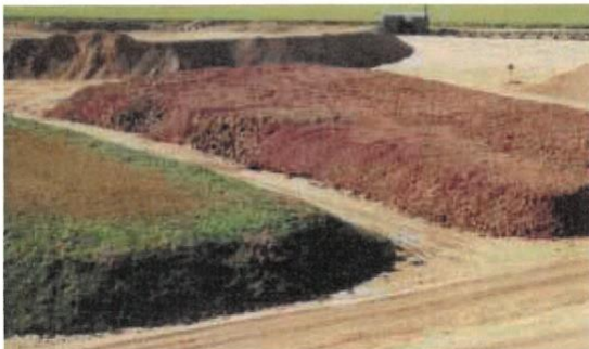
Clearly defined stockpiling of different soil materials
