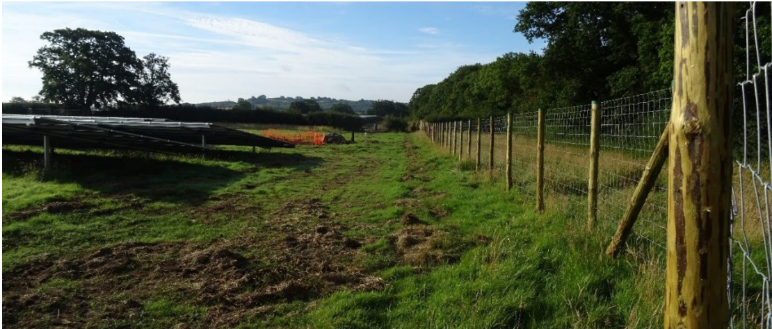
(These photos were taken on heavy, clay soils with poorly draining subsoil, and the work was photographed in July and August 2015.)
