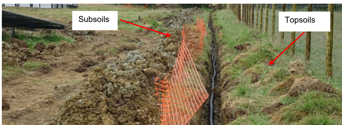
Insert 42: Subsoils Dug out of the Trench
