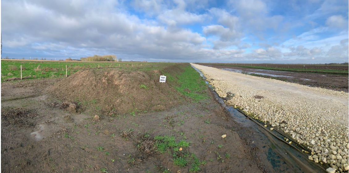
Insert 13: Temporary Topsoil Storage (January 2023)
