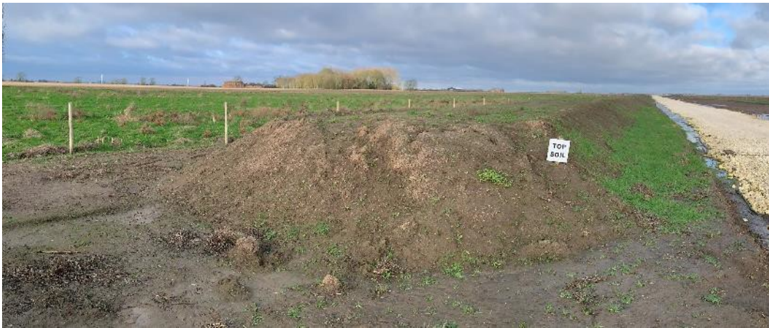
Insert 5: Temporary Topsoil Storage (January 2023)
